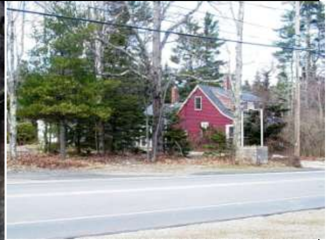
Side View of Building
