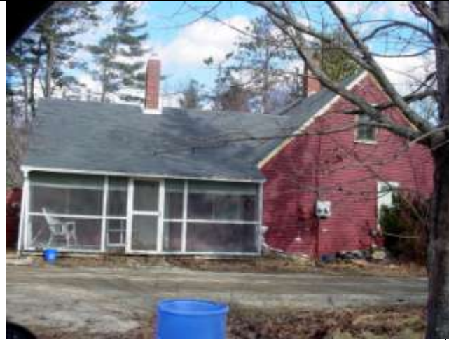
Front View of Building
